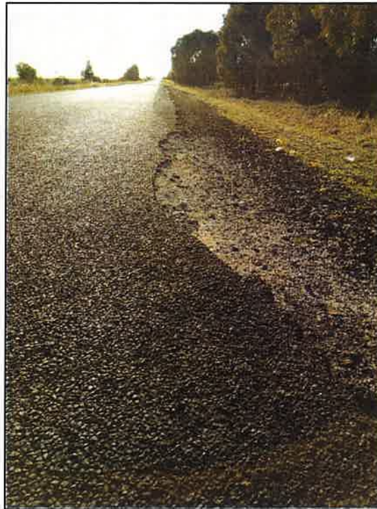
Figure 105 – Edge drop + Edge Break – Reduced Road Width (GPS: E 233765 S 6769493) W: 6.1m
