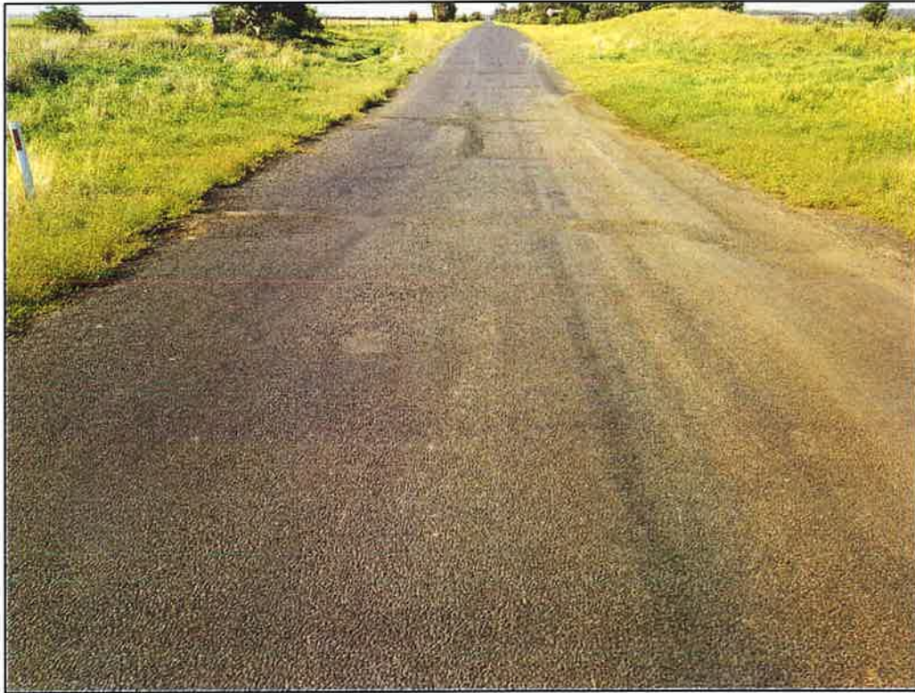
Figure 159 – Mungle Creek Floodway (pavement uneven) (GPS: E 243385, N 6790462) W:6.9m
