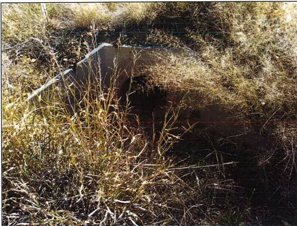
Figure 24 - Single Pipe Culvert (GPS: E 213026, S 6754353) CW: 12 W: 8.5m
