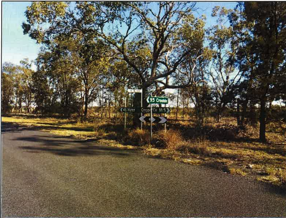
Figure 69 - Gil Gil Creek Road – Croppa Moree Road Intersection SR129 ((GPS: E 226403, S 6763002) West W: 7.1m East W: 7.05m
