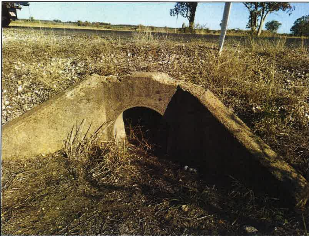
Figure 81 – Single Pipe Culvert (GPS: E 230536 S 6766552) CW: 12.4m W: 7.1m
