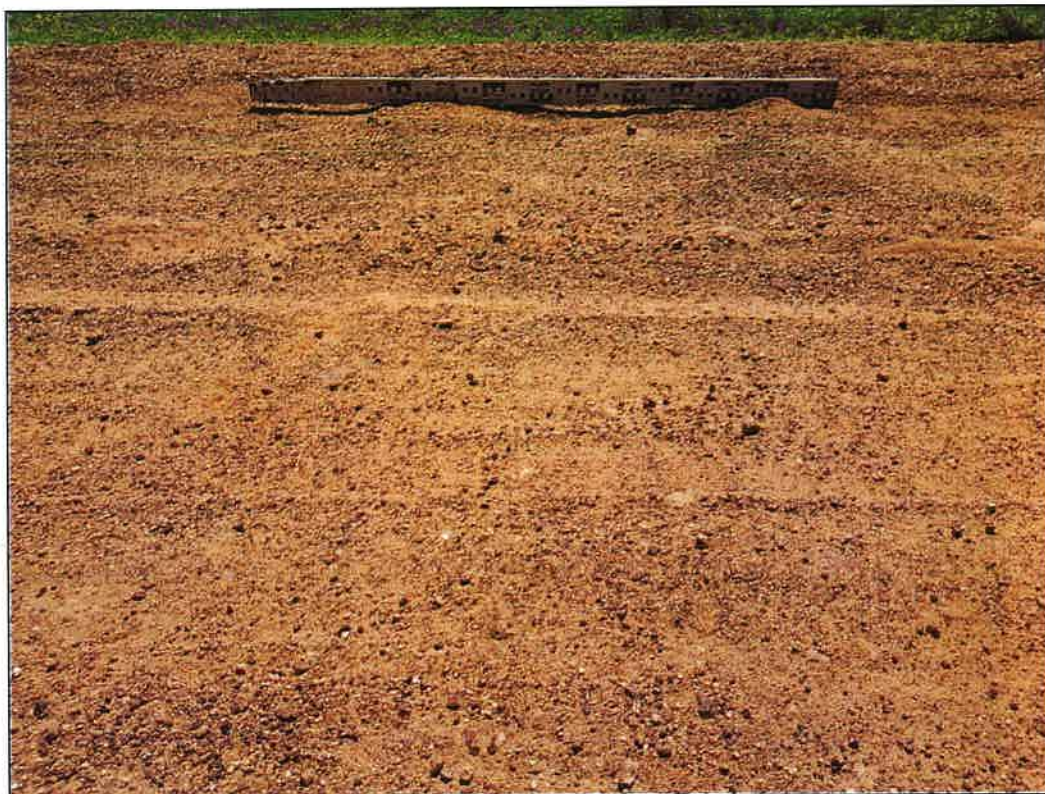
Figure 192 – Corrugation (typical to bends) (GPS: E 230905, N 6806279)
