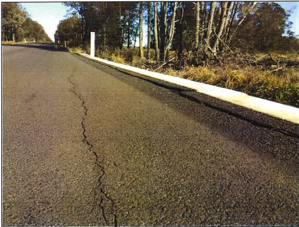
Figure 59 - Cracking on Floodway (GPS: E 225312, S6762328) L: 65.3m W: 9.25m
