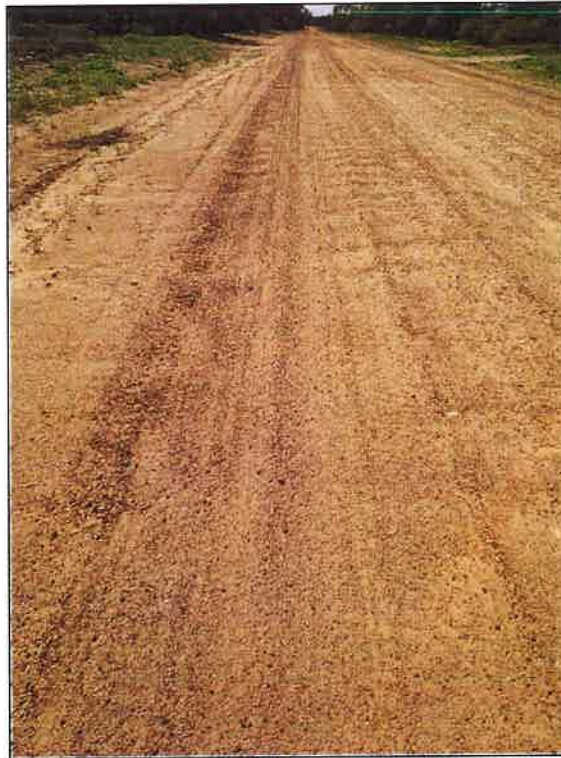
Figure 187 – I B Bore Road (Minor Corrugation) (GPS: E 229341, N 6806580)
