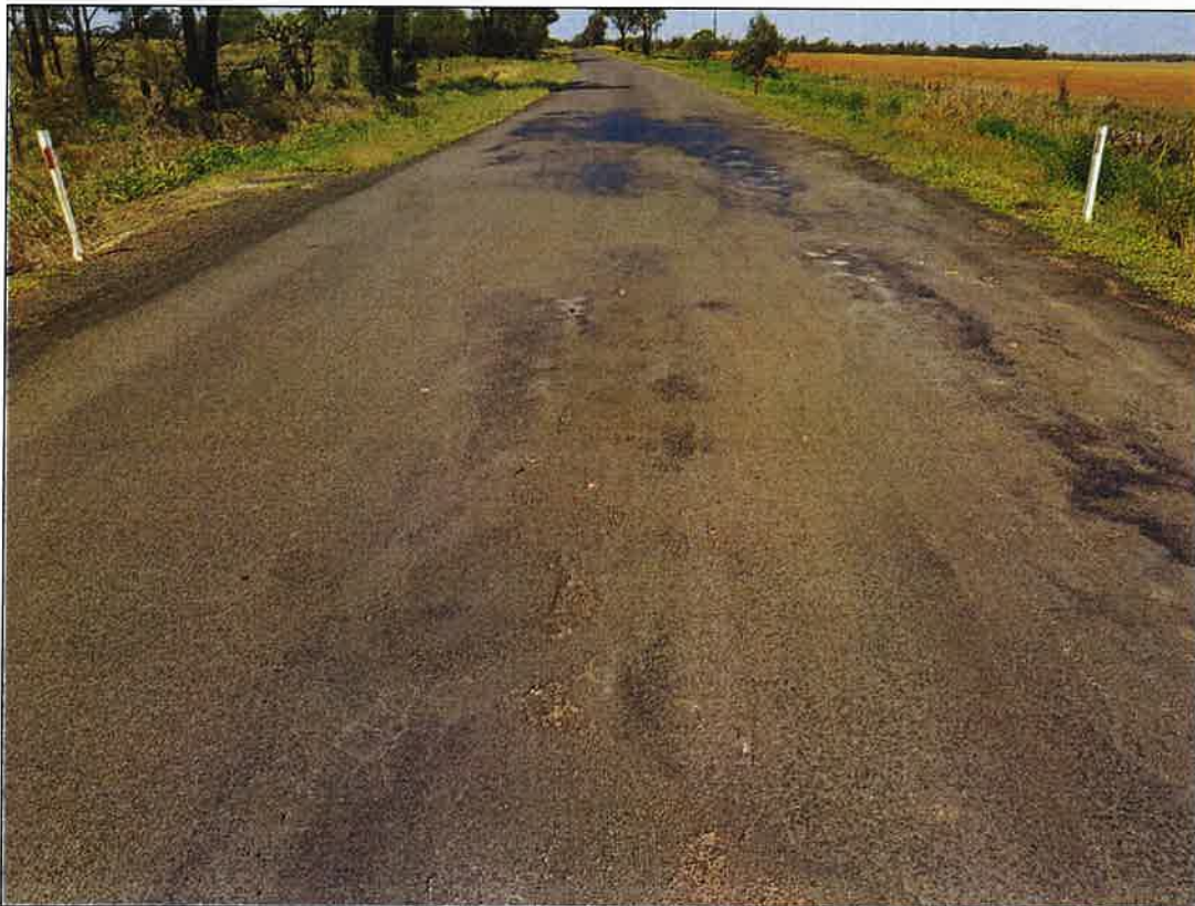
Figure 309 – Uneven Pavement
