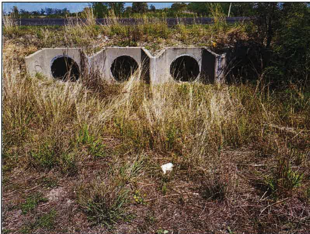
Figure 174 - Culvert Quad Pipe (GPS: E 242466, N 6783163) CW:11.4m W:7.6m
