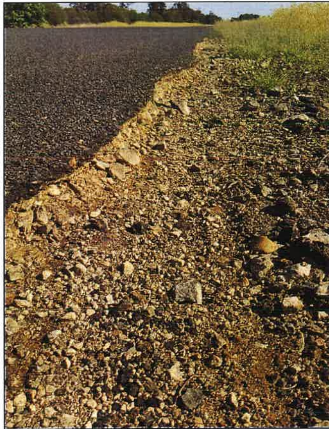
Figure 151 – Edge drop with longitudinal cracking (GPS: E 243755, N 6793282)
