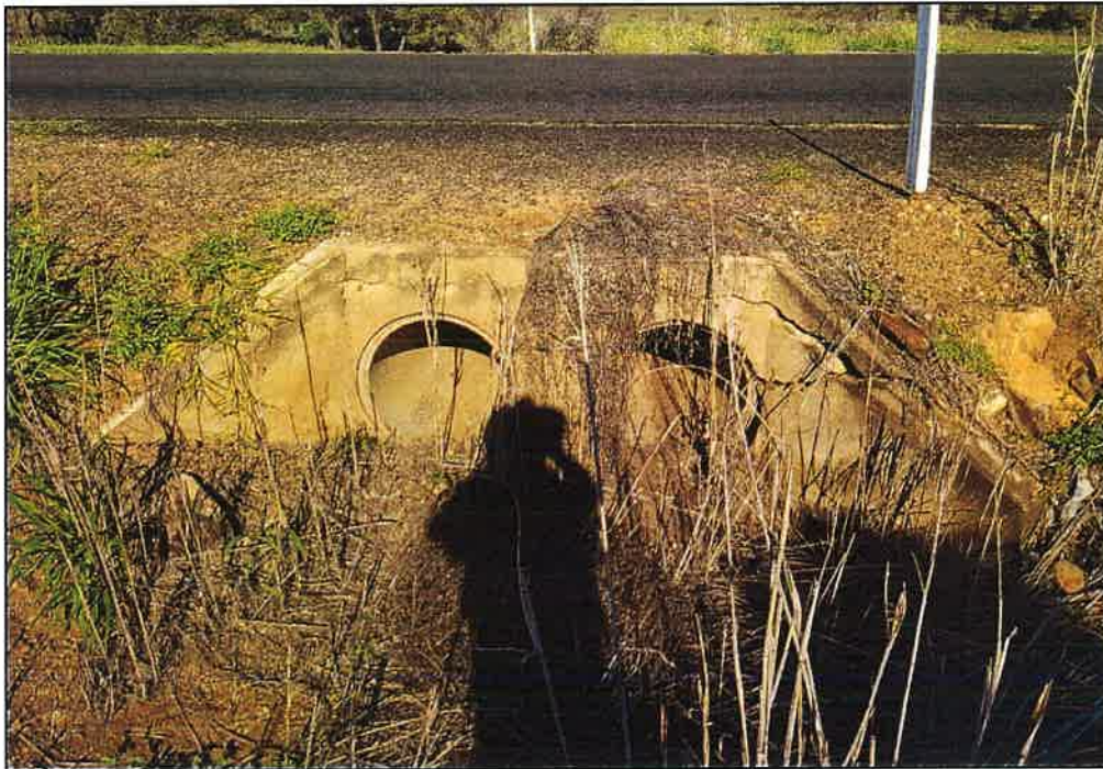
Figure 139 – Culvert Twin Pipe, Headwall Lifting Off Pipes (GPS: E 244107, N 6795956) CW: 10m W: 6.4m
