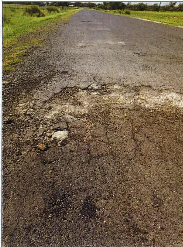
Figure 134 – Road Damage (Pothole) (GPS: E 239554, N 6773893)
