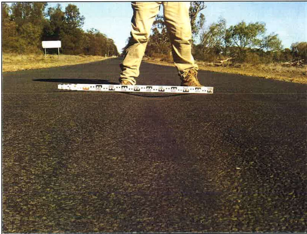
Figure 63 – Moderate Rutting (GPS: E 225578, S 6762489)
