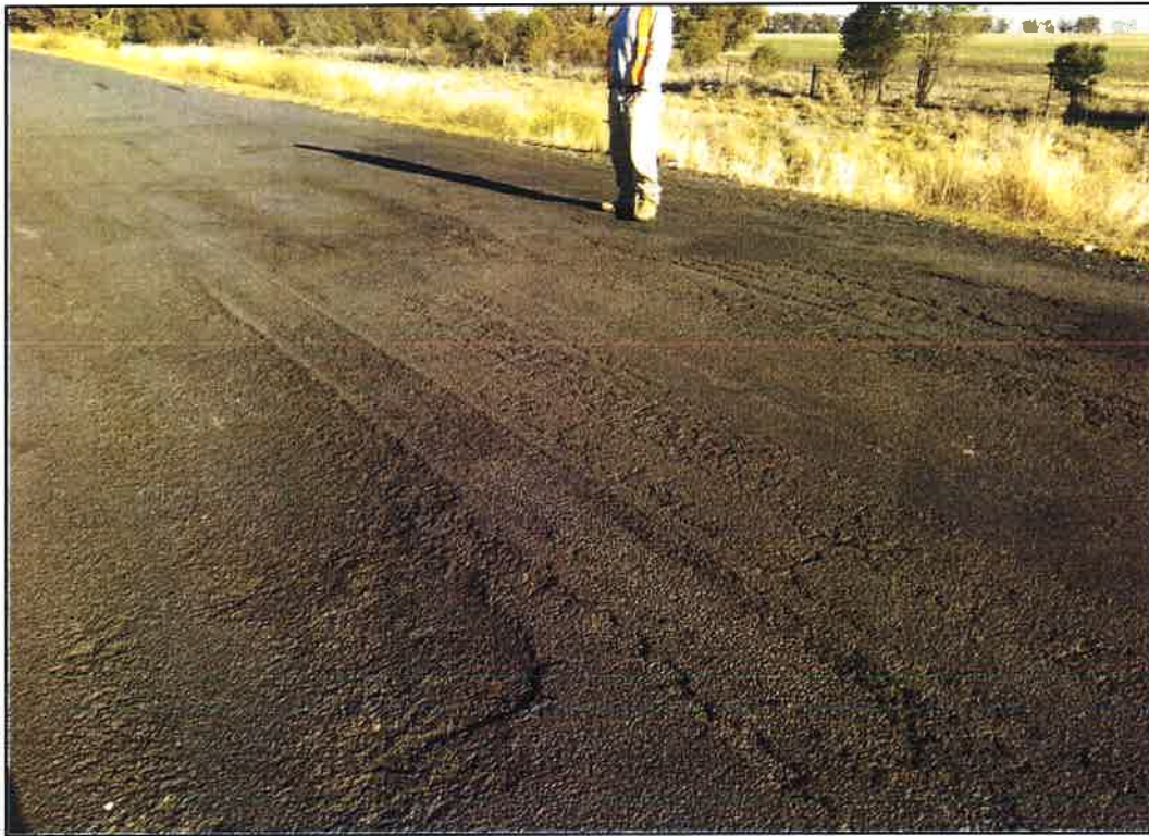
Figure 107 – Patchwork and Rutting above Triple Pipe Culvert (GPS: E 235519 S 6770828) CW: 10.1 W: 7m
