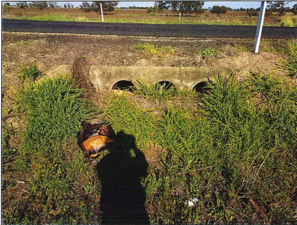
Figure 143 - Culvert Quad Pipe (GPS: E 244010, N 6795231) CW: 9.9m W: 6.5m
