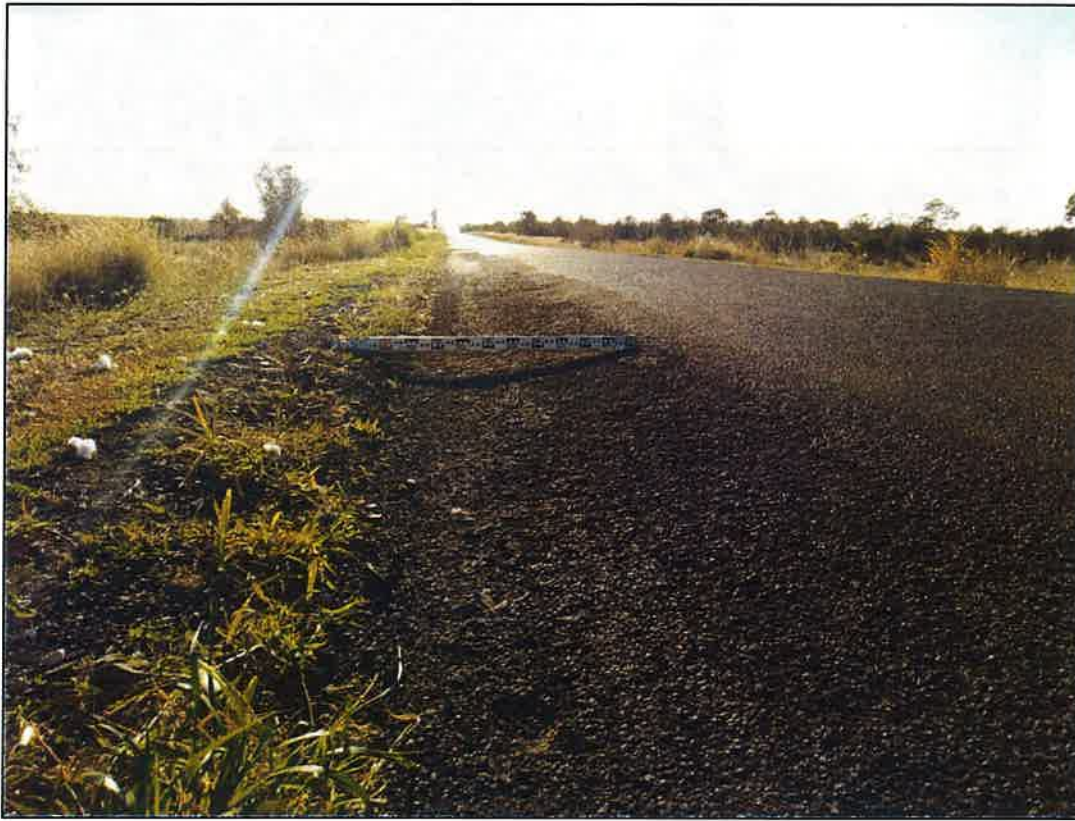
Figure 113 – Rilling above Single Pipe Culvert (GPS: E 233519 S 6770828)
