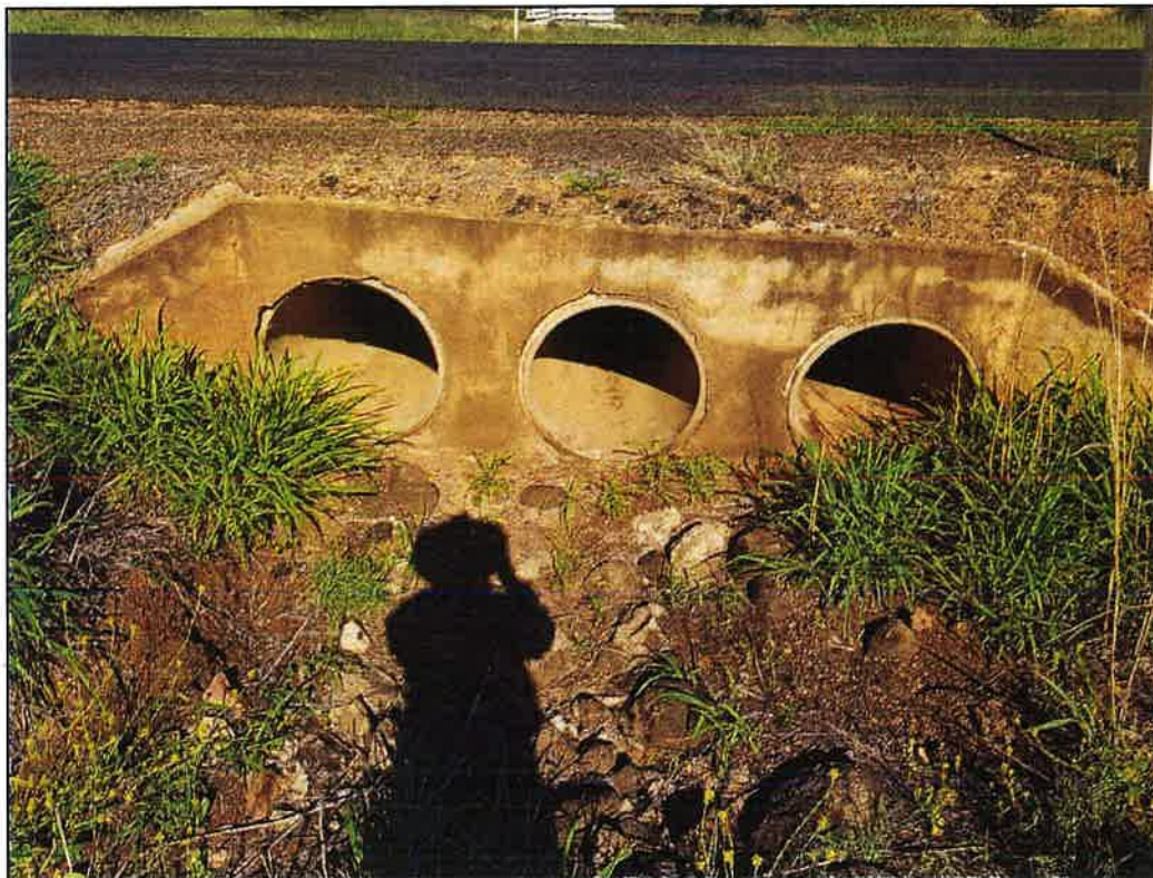
Figure 148 – Culvert Triple Pipe (GPS: F 243923, N 6794560) CW: 12.6m W: 6.4m
