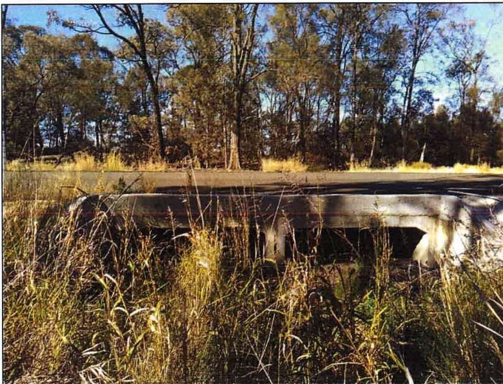
Figure 60 - Floodway Twin Box Culvert (GPS: E 225312, S6762328) L: 65.3m W: 9.25m
