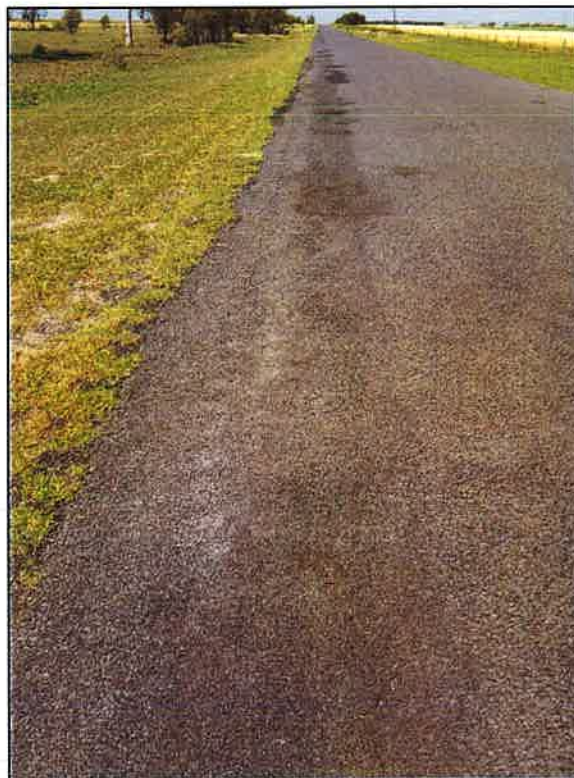
Figure 180 – Localised edge break, vegetation growing through shoulder (GPS: E 242242, N 6781714)
