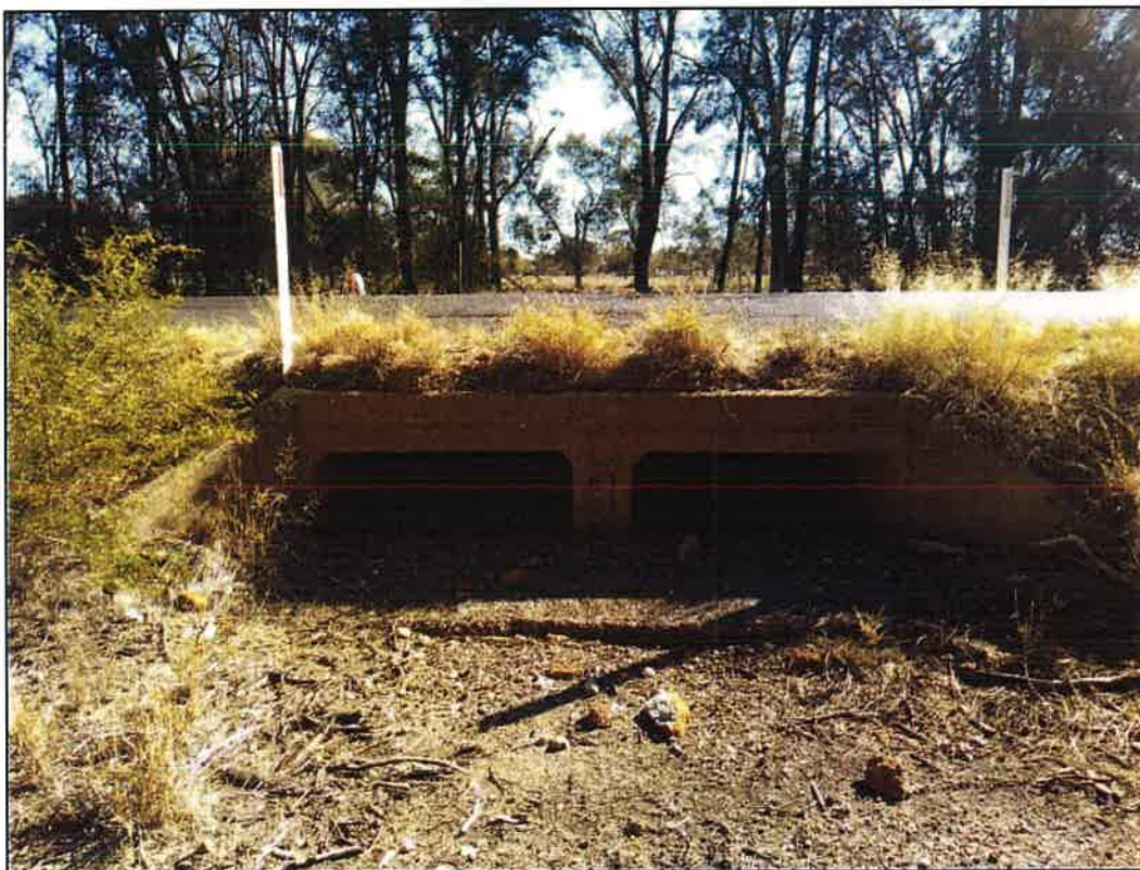
Figure 44 - Twin Box Culvert - Patchwork and minor rutting above (GPS: E 221555, S 6760081) CW: 10.2m W: 7.3m
