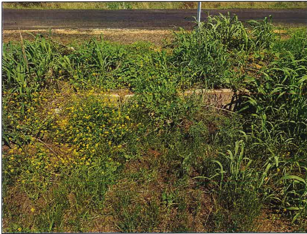
Figure 167 - Culvert Twin Pipe - Blocked (GPS: E 242768, N 6785708) CW:11.5m W:6.7m
