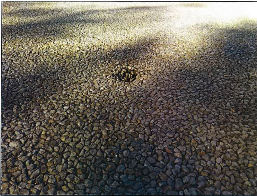
Figure 53 – Pothole above Single Pipe Culvert (GPS: E 224434, S 6761722) CW: 10m W: 7.4m
