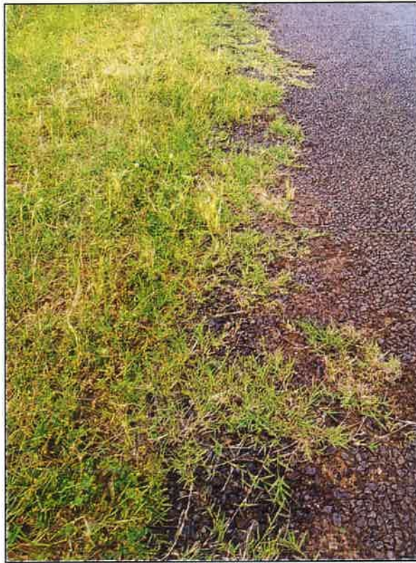
Figure 270 – Edge break (GPS: E 244769, N 6796804)
