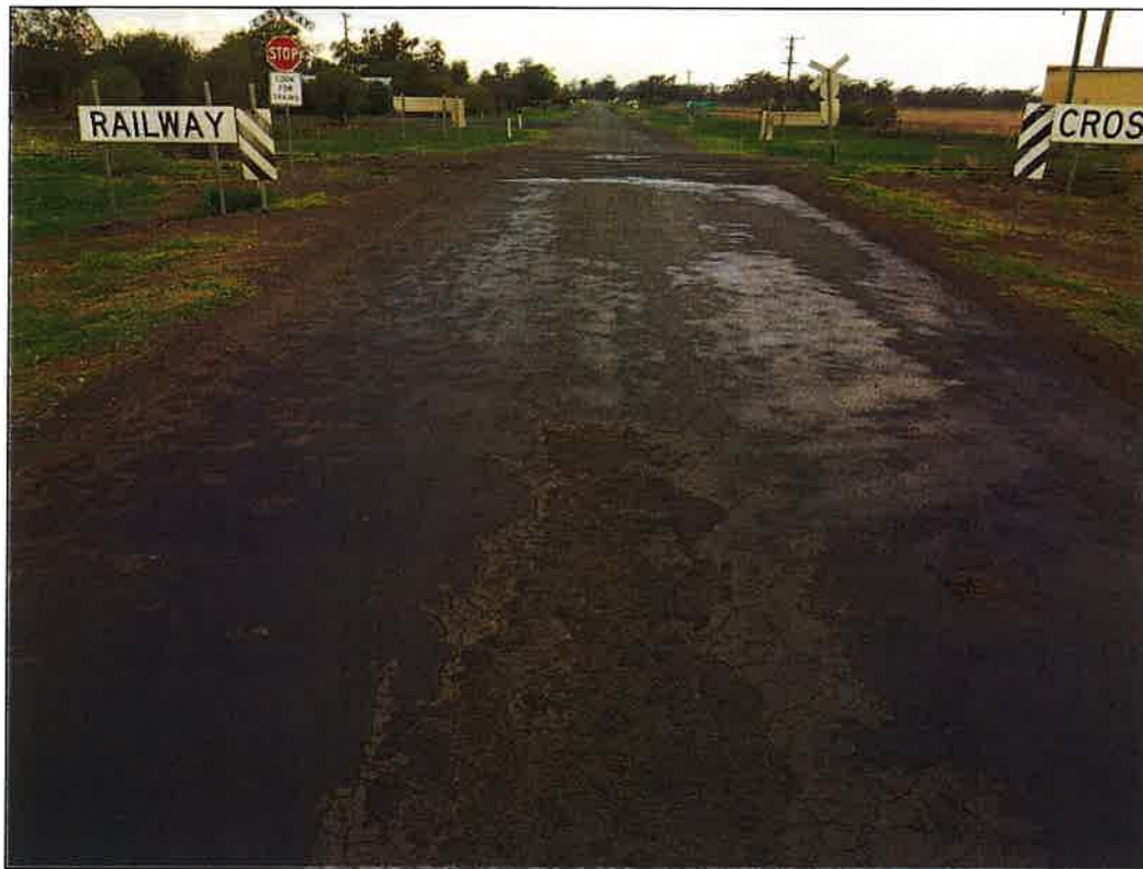
Figure 276 – Railway Crossing (Spider Cracking) (GPS: E 245624, N 6796687) W:5.4m
