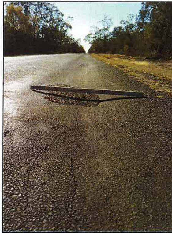
Figure 49 – Rutting and Patchwork (GPS: E 222167, S 6760496)
