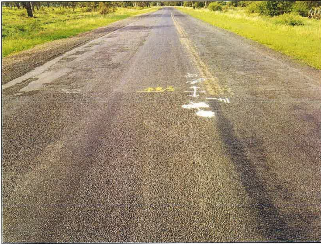
Figure 342 - Bruxner Way Section Change (Road damage for approx 100m) (GPS: E 247038, N 6826914) W:7.8m
