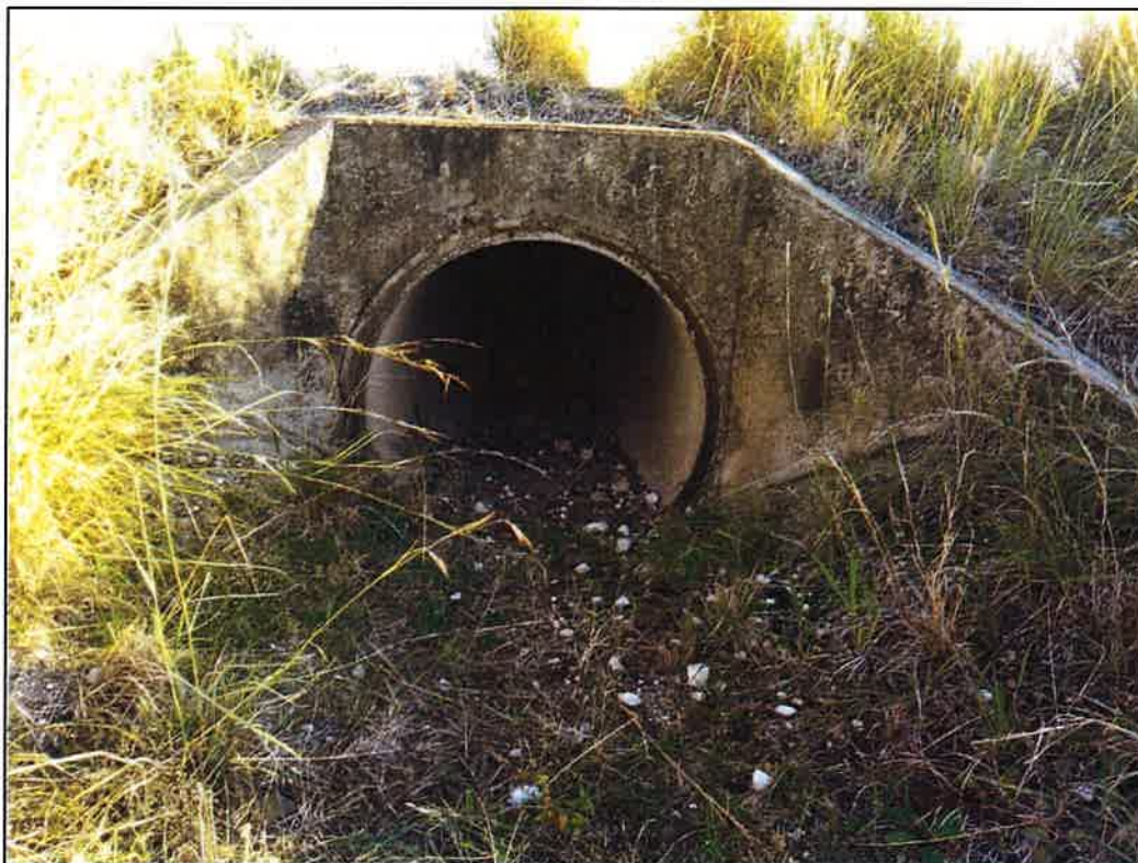
Figure 110 - Single Pipe Culvert (GPS: E 233519 S 6770828) CW: 10.2 W: 7m
