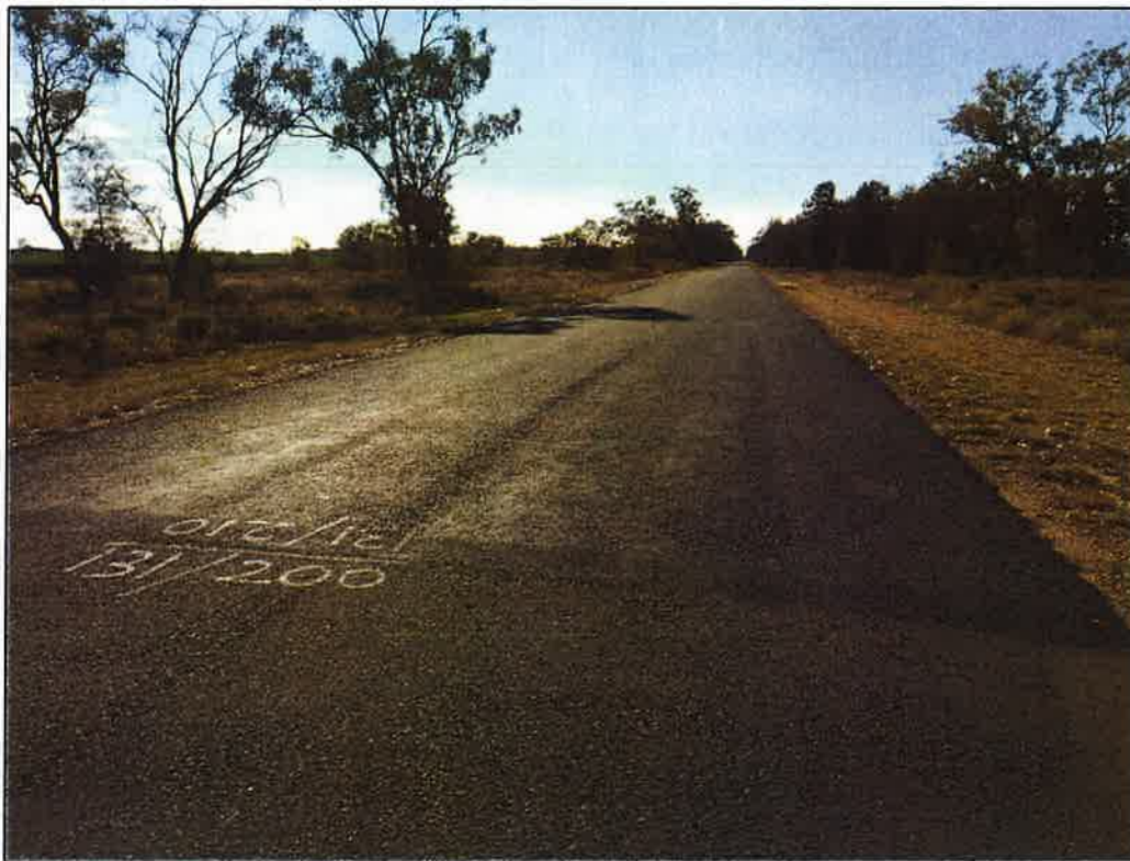
Figure 61 - Section Change (GPS: E 225312, S6762328) East W: 7.2m, West W: 8.1m
