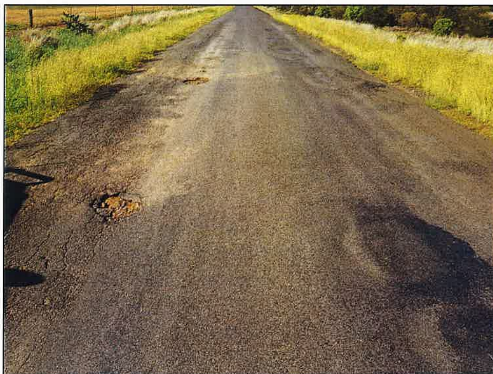
Figure 154 – Potholes, cracking and shoving (GPS: E 243651, N 6792465)
