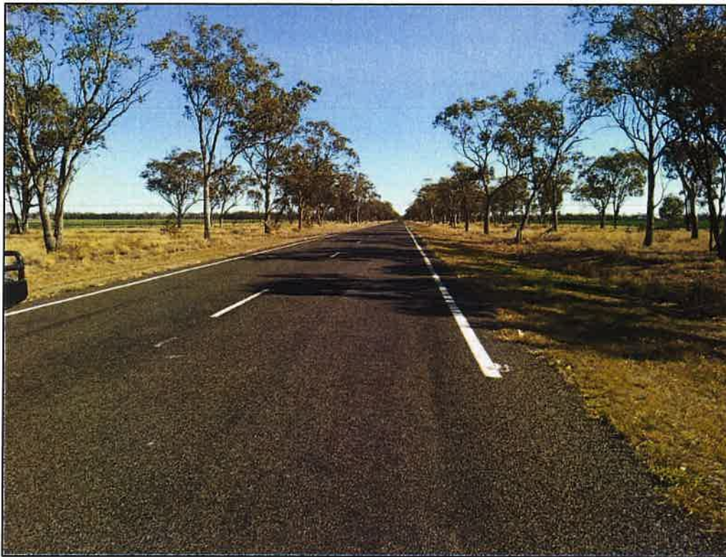
Figure 21 – Section Change: End of Shoulder Line Marking (GPS: E 210808, S 6754450) W: 8.4m
