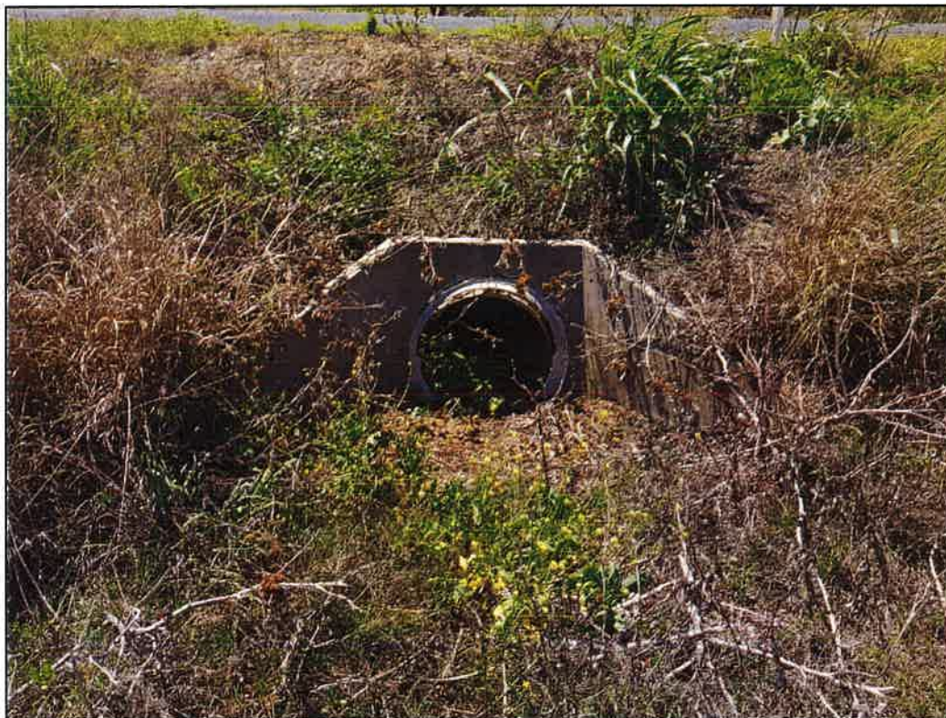
Figure 184 – Culvert Single Pipe (GPS: E 240764, N 6779468) CW: 12.1 W:4.3m
