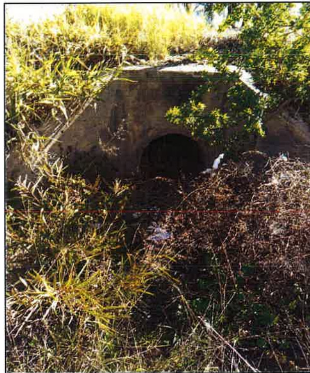
Figure 52 – Single Pipe Culvert (GPS: E 224434, S 6761722) CW: 10m W: 7.4m
