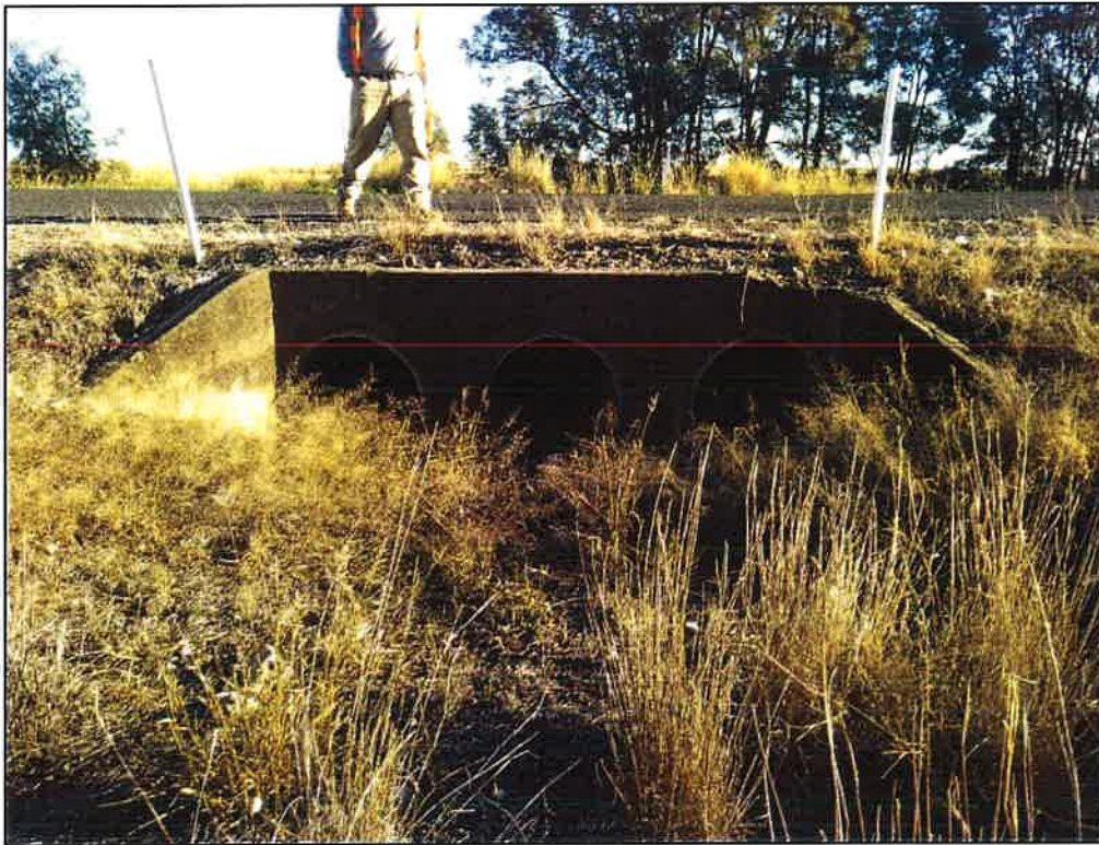
Figure 115 – Triple Pipe Culvert (GPS: E 233519 S 6770828) CW: 10.2m W: 7.5m
