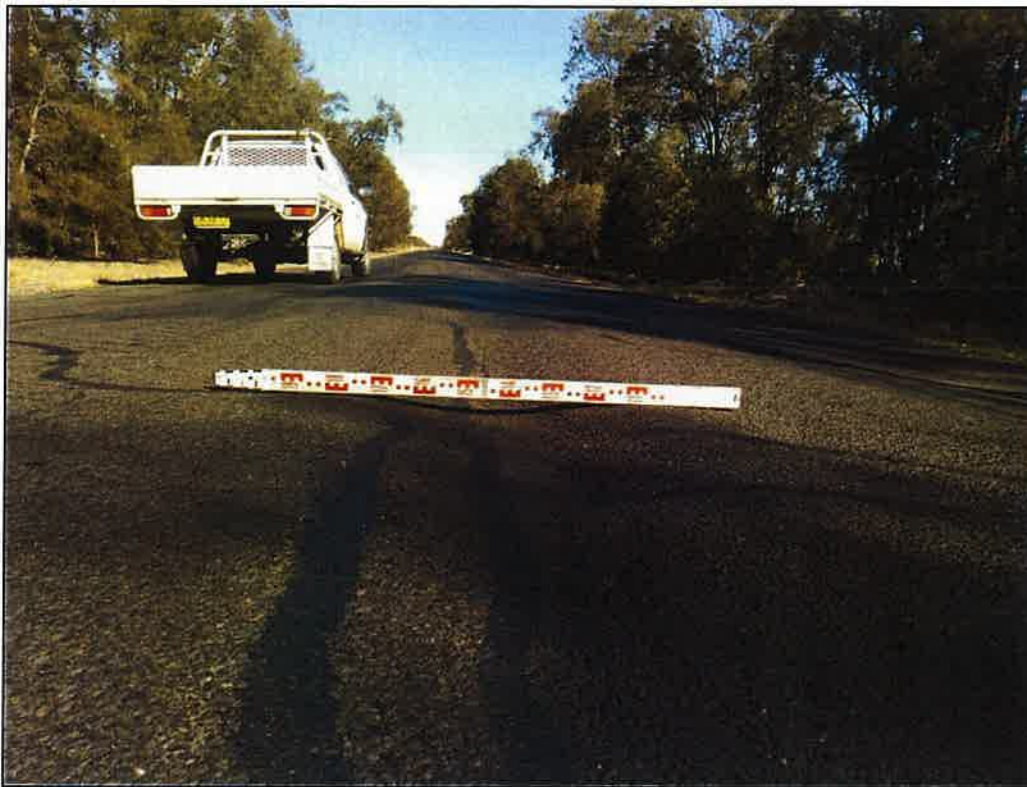
Figure 45 – Rutting and Patching (GPS: E 221555, S 6760081)
