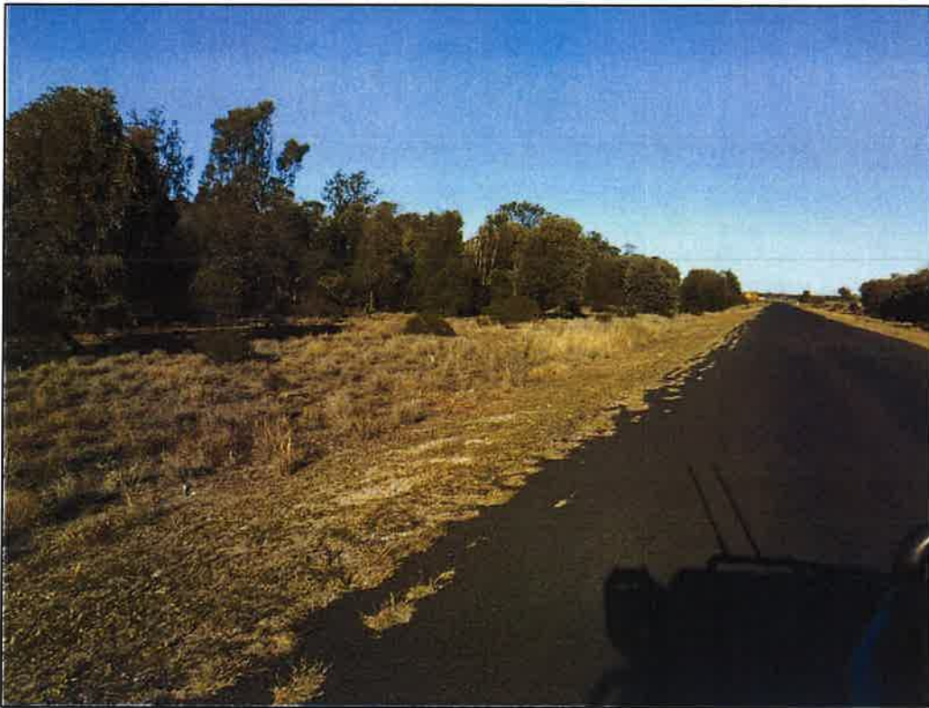
Figure 93 - Vegetation growth through bitumen shoulders causing edge break (GPS: E 231002 S 6767395) W: 6m
