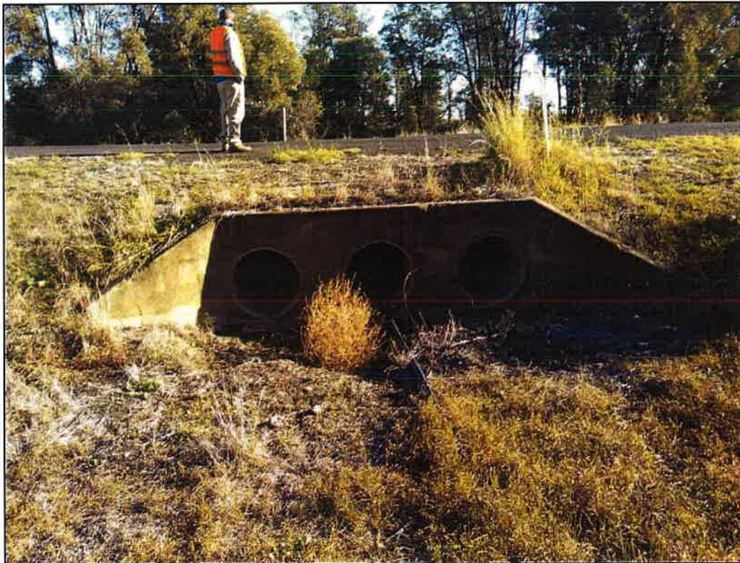
Figure 104 – Triple Pipe Culvert (GPS: E 233765 S 6769493) CW: 12.6 W: 7m
