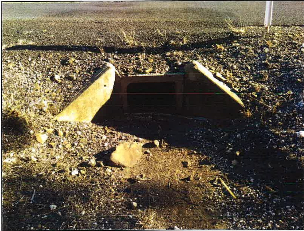
Figure 99 – Single Box Culvert (GPS: E 231958 S 6768126) CW: 9.6m RW: 6.75
