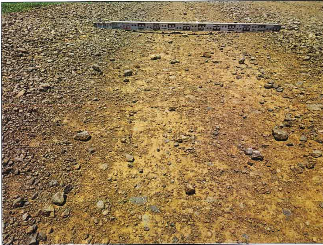
Figure 235 – Typical Minor Rutting (GPS: E 239493, N 6800359)
