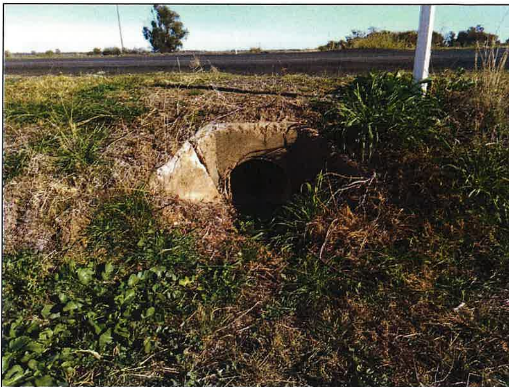
Figure 82 - Single Pipe Culvert (GPS: E 230684 S 6767141) CW: 10.4m W: 6m
