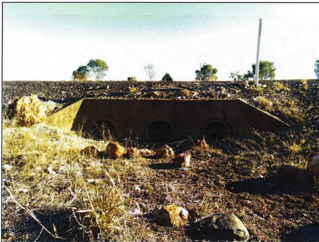
Figure 106 - Triple Pipe Culvert (GPS: E 235519 S 6770828) CW: 10.1 W: 7m
