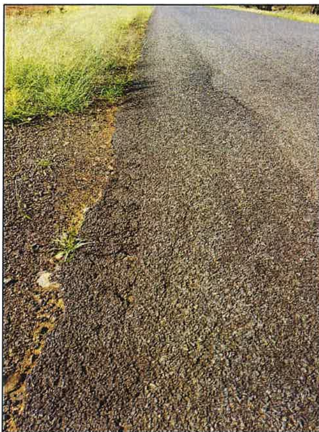
Figure 153 – Patched edge work (GPS: E 243651, N 6792465)
