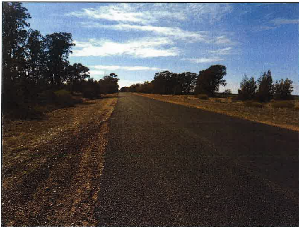
Figure 42 – Westbound Traffic has a Depression on the Southern Edge of the Road (GPS: E 220359, S 6759281) W: 7m
