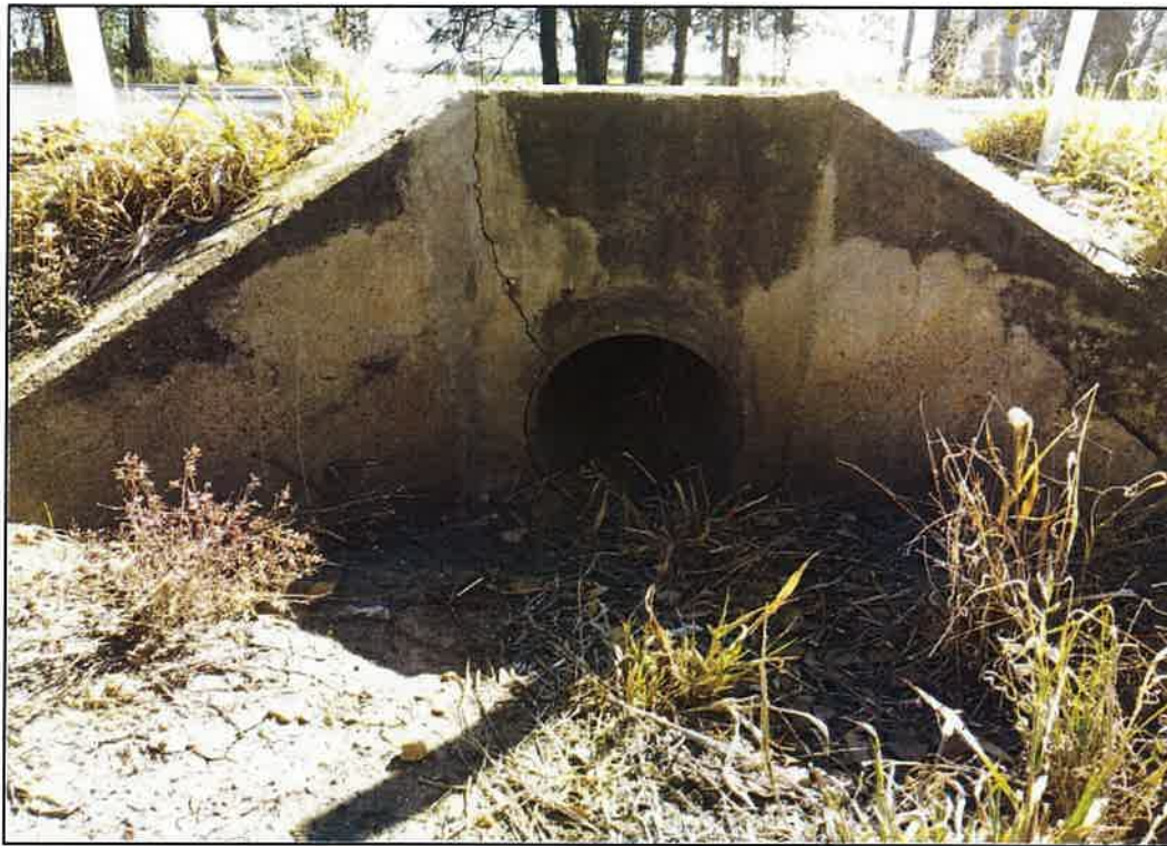
Figure 25 – Single Pipe Culvert (GPS: (GPS: E 213955, S 6754961) CW: 10 W: 7.9m
