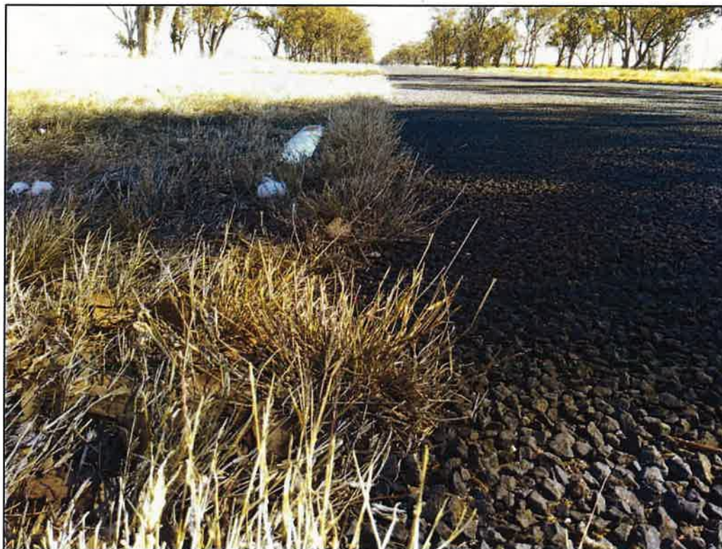
Figure 22 – Vegetation growing through the bitumen (mainly westbound lane)
