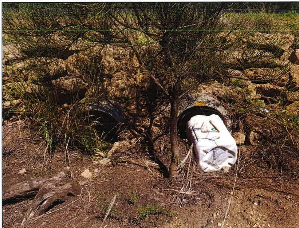
Figure 168 - Culvert Twin Pipe (GPS: E 242732, N 6785454) CW:14.4m W:7.7m
