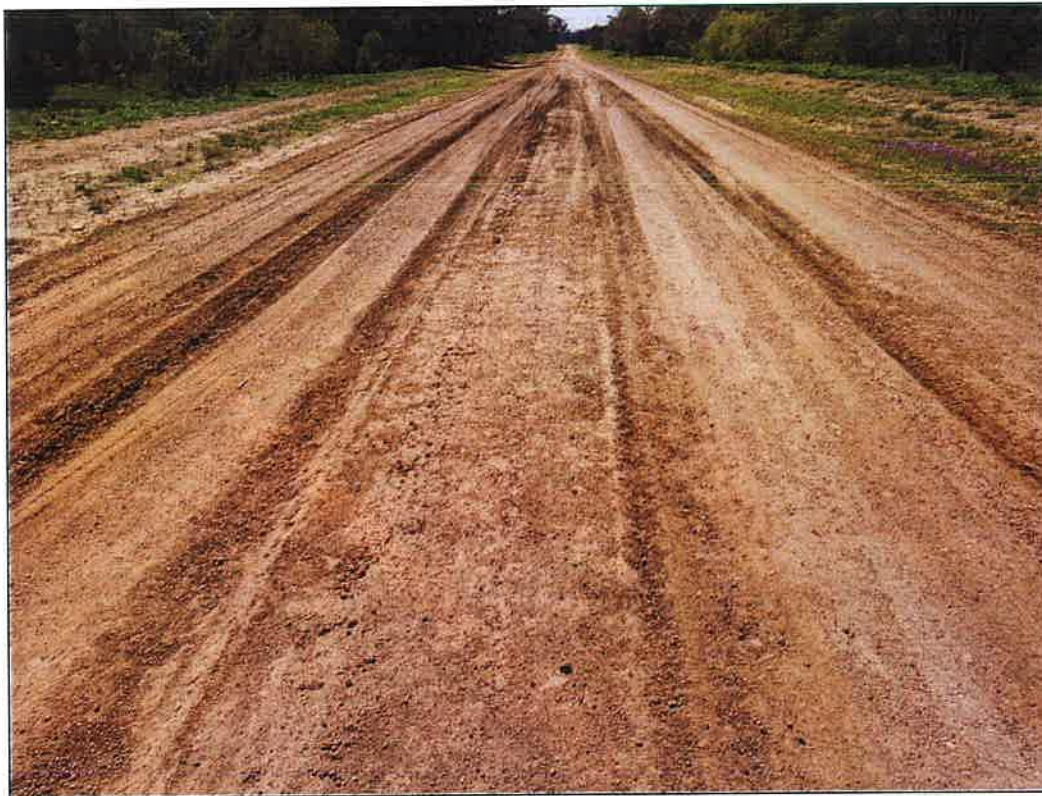
Figure 188 – Gravel Wearing Thin to Dirt (GPS: E 229568, N 6806544) W:6.8m
