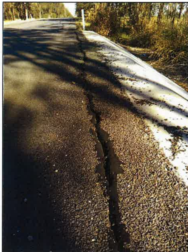
Figure 58 - Edge Drop on Floodway (GPS: E 225312, S6762328) L: 65.3m W: 9.25m
