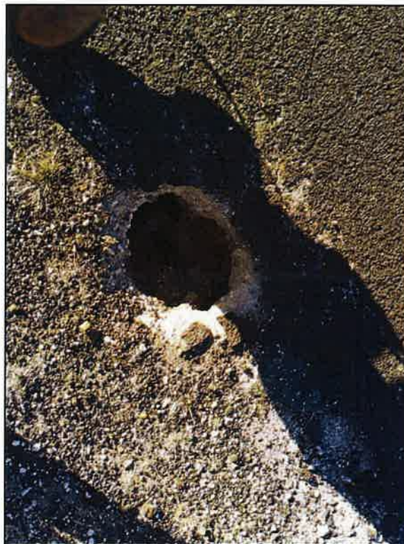
Figure 94 - Significant Pot Hole through to Culvert (GPS: E 231002, S 6767395)
