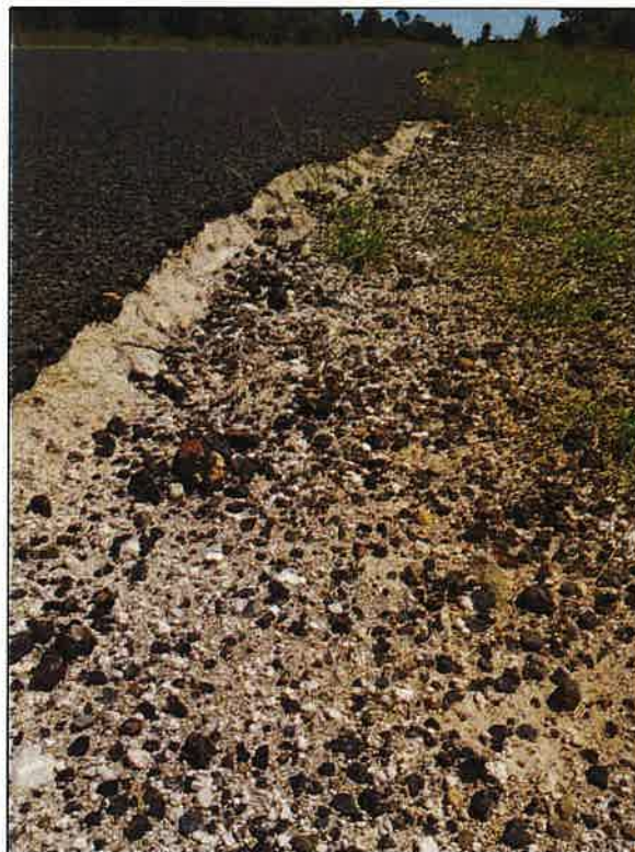
Figure 126 – Edge Drop (GPS: E 236981, N 6771917) W:6.6m
