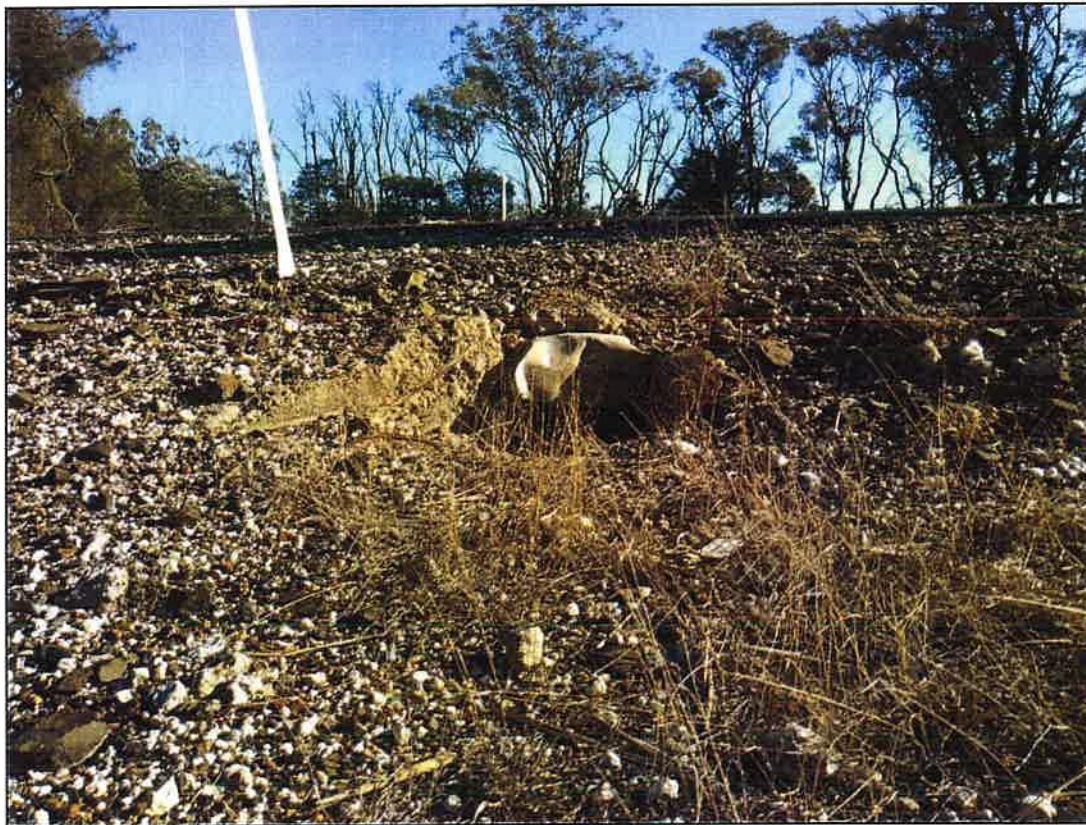
Figure 95 – Single Pipe Culvert – Collapsed with Spider Cracking on Road (GPS: E 231002, S 6767395) CW: 10.1m W: 6.6m
