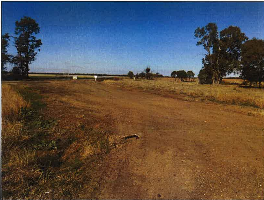
Figure 54 – Double Property Access “Glenelg” – Approx. 300m Sight Distance to West (GPS: E 224433, S 6761752) W: 7.2m
