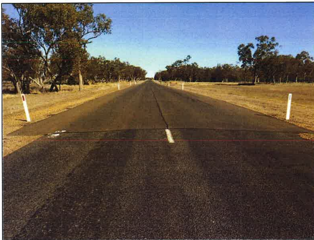
Figure 36 - Section Change - End of Floodway (GPS: E 218248, S 6757831) East RW: 7.3m, West RW: 9.2m
