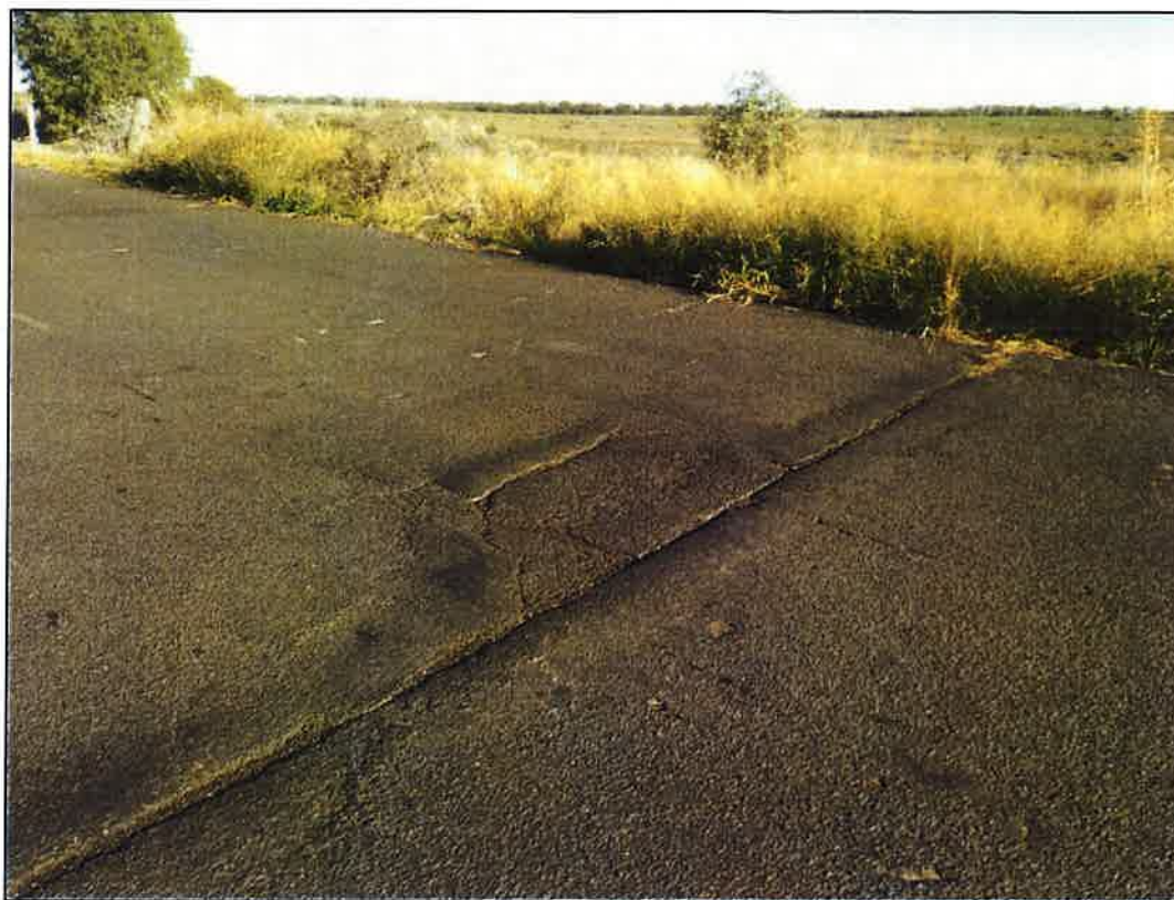
Figure 97 – Causeway – Expansion Joint (GPS: E 231879, S 6768062) W: 7.2m (narrow) Length: 40m
