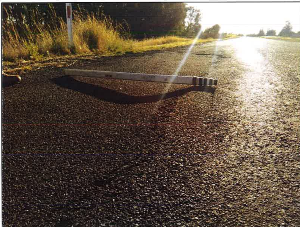
Figure 116 - Triple Pipe Culvert (Rutting and Rilling above Culvert) (GPS: E 233519 S 6770828) CW: 10.2m W: 7.5m
