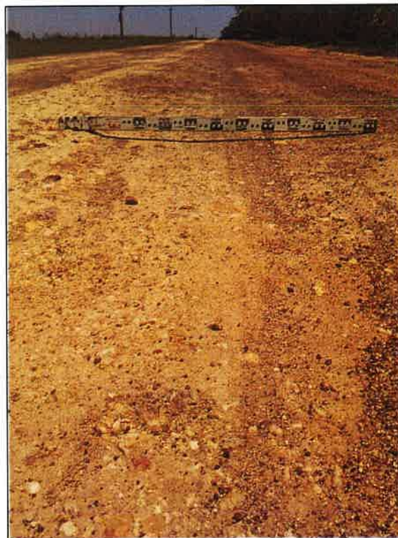
Figure 212 – Rutting, generally minor (GPS: E 232239, N 6801346)
