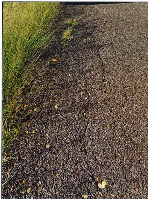
Figure 150 – Minor edge break with vegetation growing through shoulder (GPS: E 243818, N 6793760)
