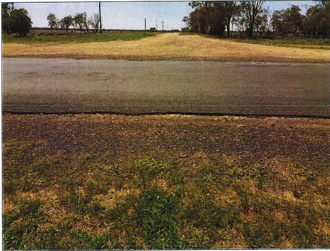
Figure 310 – Property Access (Localised Edge Drop)
