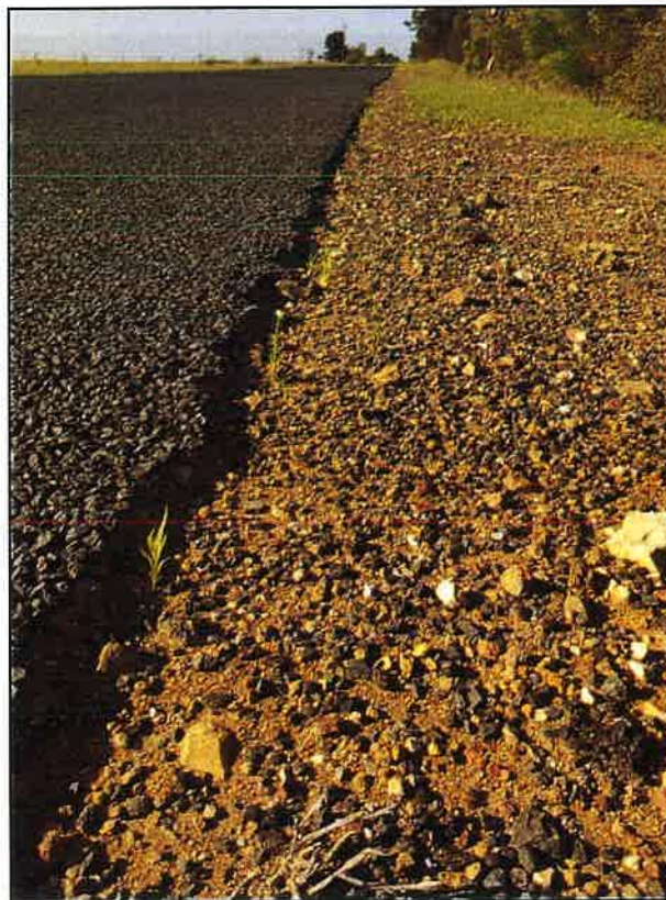
Figure 140 – Edge Drop (GPS: E 244107, N 6795956)
