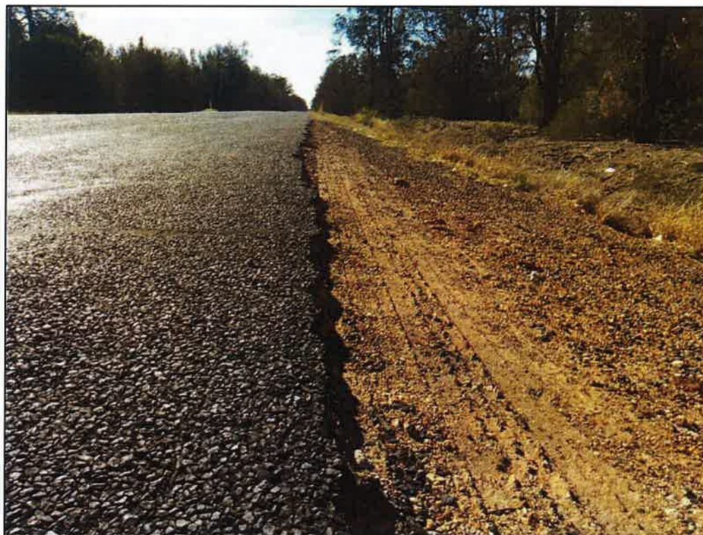
Figure 46 – Edge Drop (GPS: E 221555, S 6760081)
