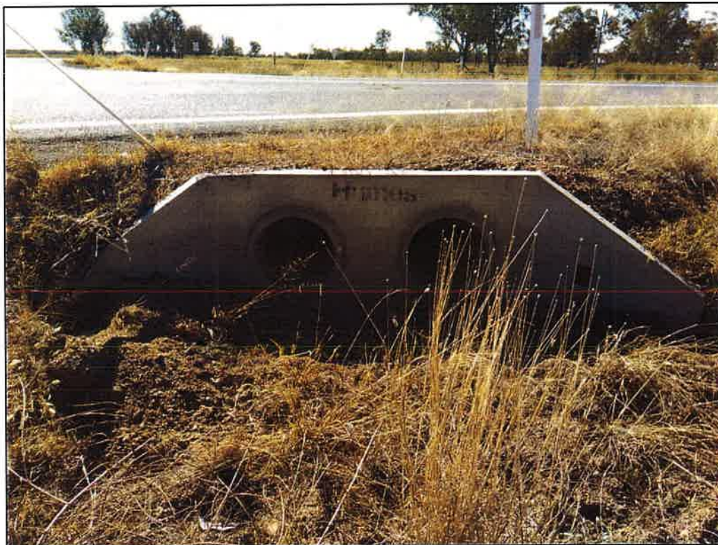
Figure 16 – Culvert Twin Pipe (GPS: E 789696, N 6754883) CW: 12.10 W:8.5m
