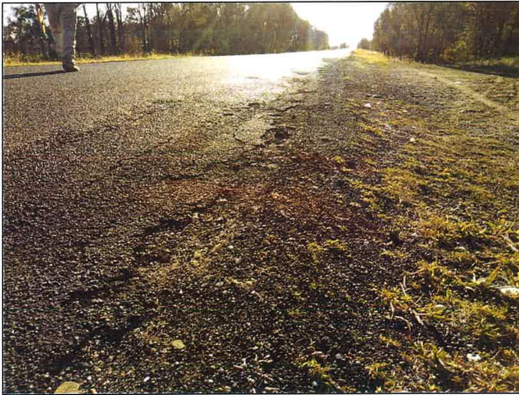
Figure 103 – Minor Edge Break at Dual Property Access (GPS: E 233765 S 6769493) W: 6.9m
