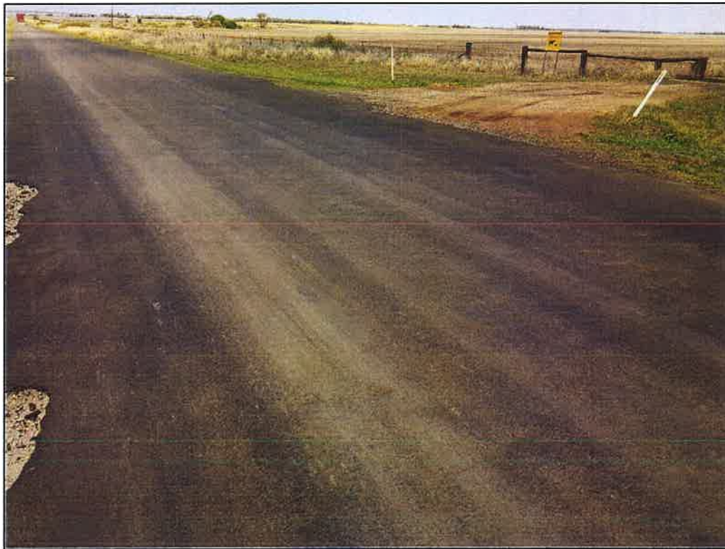
Figure 183 – Tumba Road Intersection with Croppa Creek Road (localised edge break) (GPS: E 241989, N 6779852) W:6.6m
