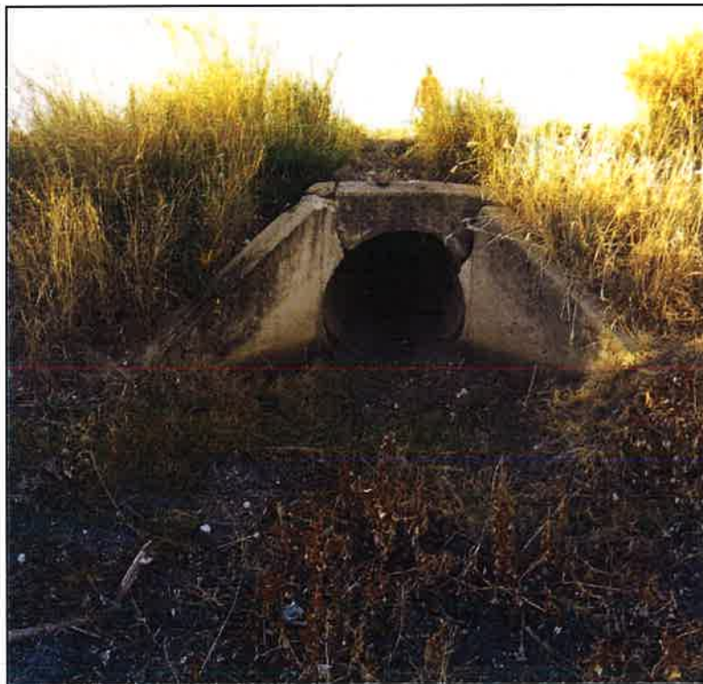
Figure 112 – Single Pipe Culvert – Head Wall Damage (GPS: E 233519 S 6770828) CW: 12.9m W: 7m
