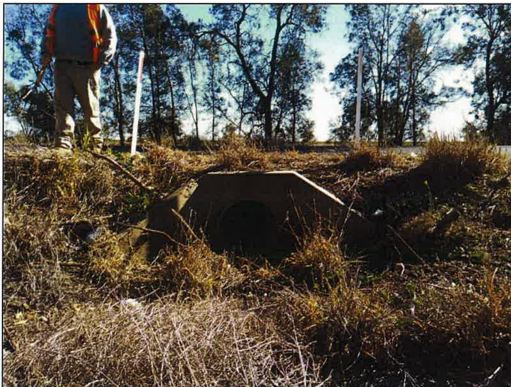
Figure 62 – Single Pipe Culvert (GPS: E 225578, S 6762489) CW: 9.8m W: 7.2m
