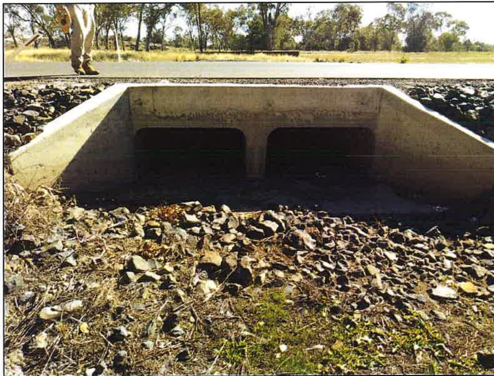
Figure 35 – Twin Box Culvert (Floodway) (GPS: E 218248, S 6757831) CW: 12.40m, W: 9.10m
