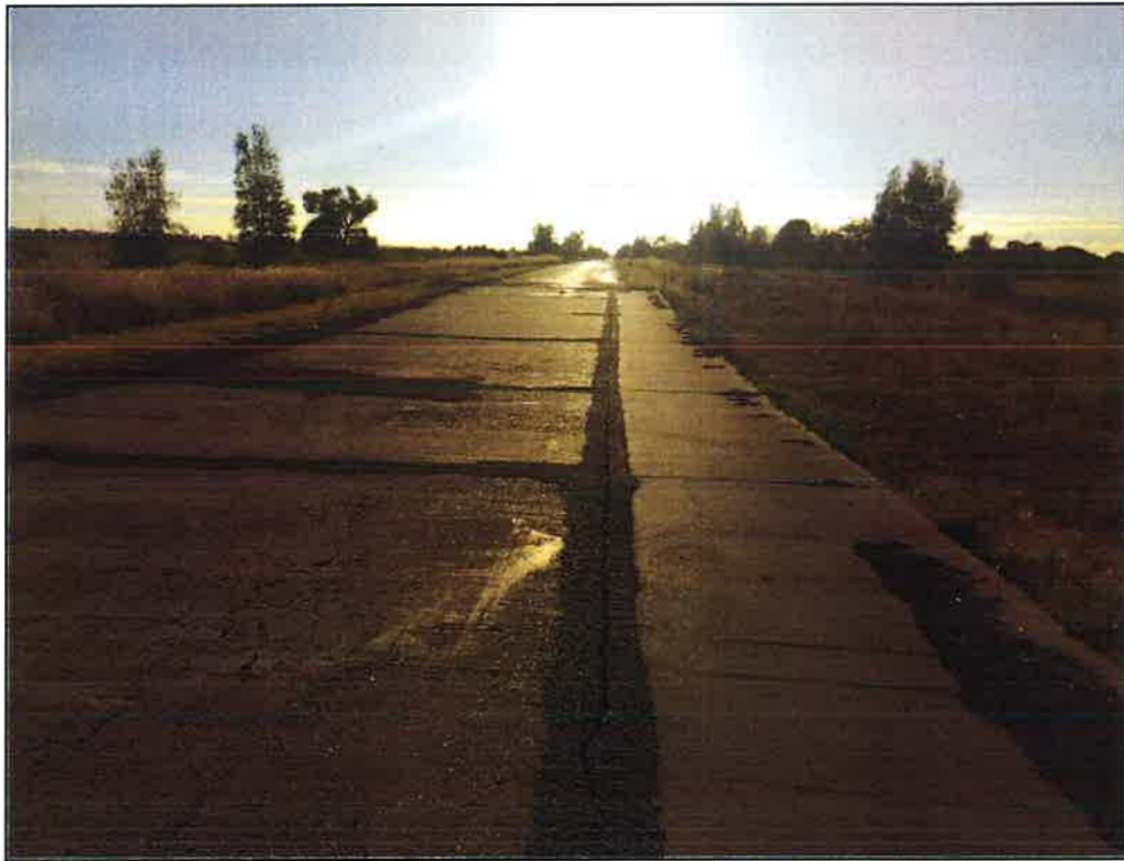
Figure 119 Floodway – Patched – Speed Limit 65km/h (GPS: E 236528 S 6771621) Length: 39.85m W: 9m
